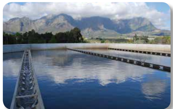
Treated effluent produced from an AquaNereda® reactor.
